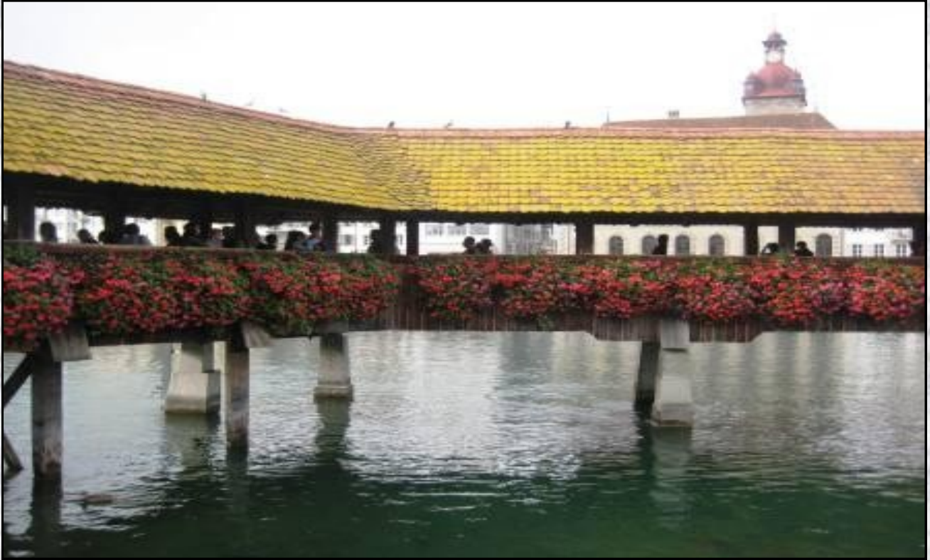
One of the wooden bridges at Luzerne.
